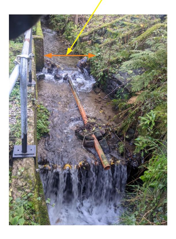
the dam can be fixed to the concrete on the nearside bank. For the far side we will need to fix a concret post or similar into the river bed, here;
